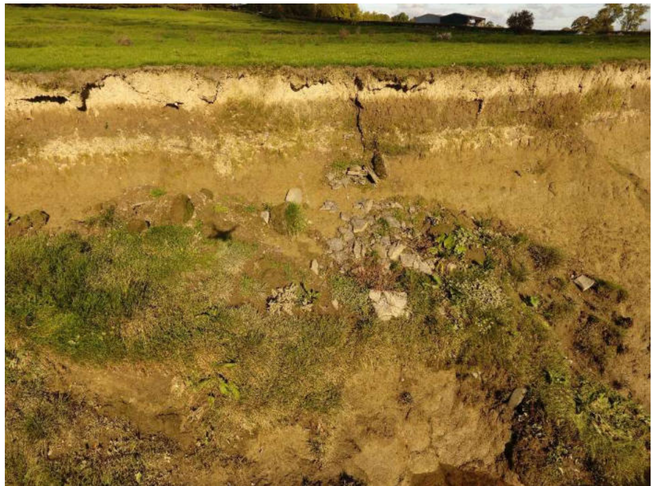
Fig. 12. Erosion of bank of River Severn at Strata Marcella
